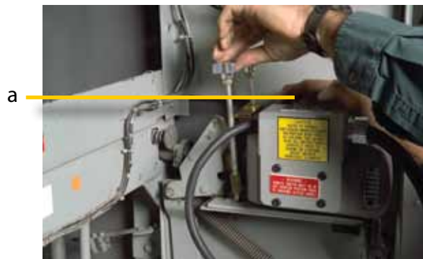
Figure 4 Mechanism Keeper Arm in Place
