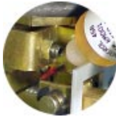
c. Trip Shaft Bearing
