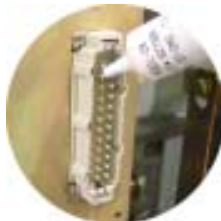
b. Secondary Disconnect Receptacle
