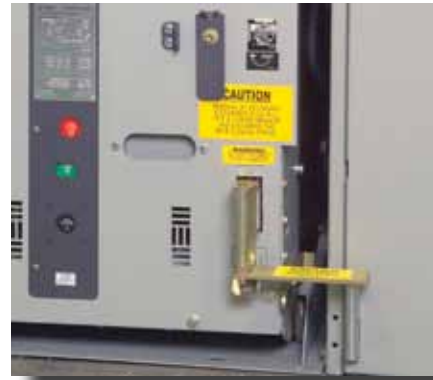
Figure 11 Secondary Disconnect Override Device
