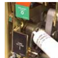
ac. Motor Cutoff Cam
