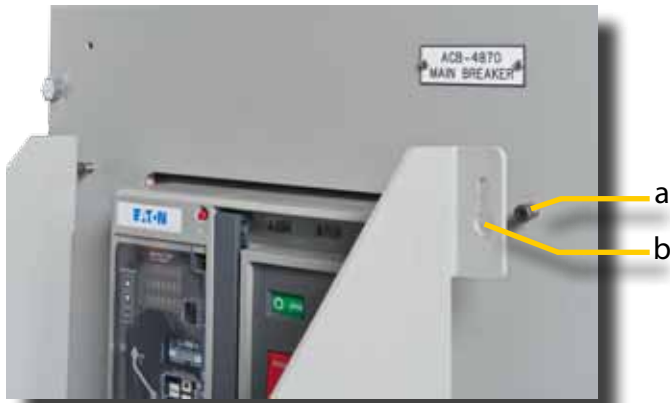
Figure 3 Positioning RRD onto LV Switchgear
