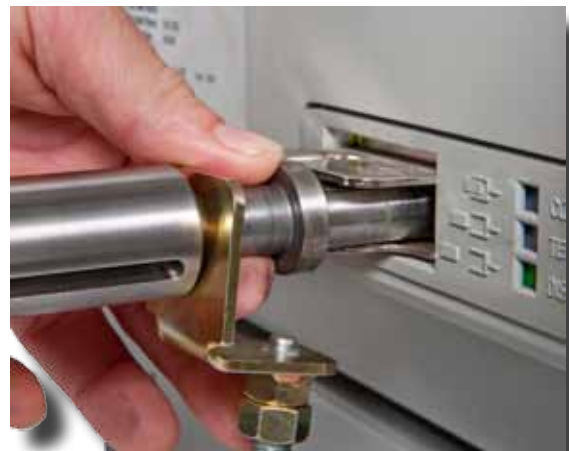
Figure 6 Engaging Racking Shaft
