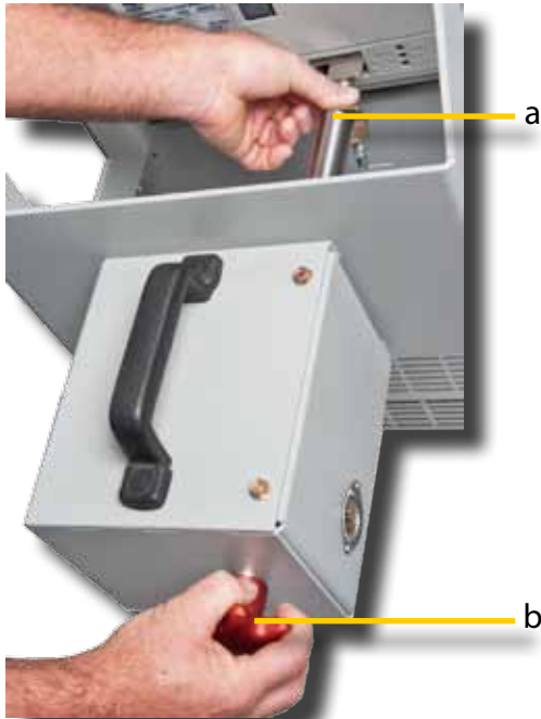
Figure 7 Aligning Racking Shaft
