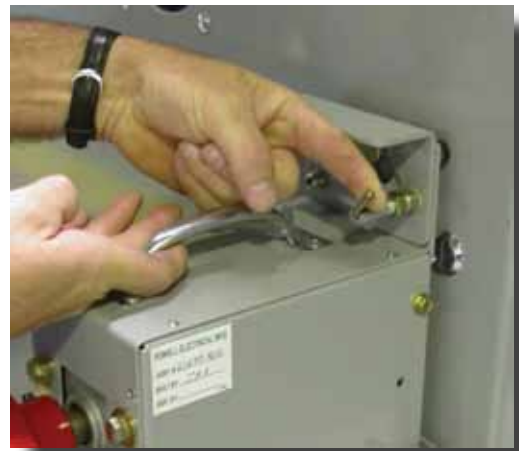
Figure 16 Unlatch the Racking Device Spring Lock Pin
