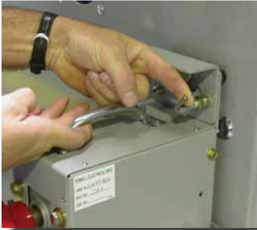
Figure 9 Insert the Drive Socket into the Racking Shaft Access Opening
