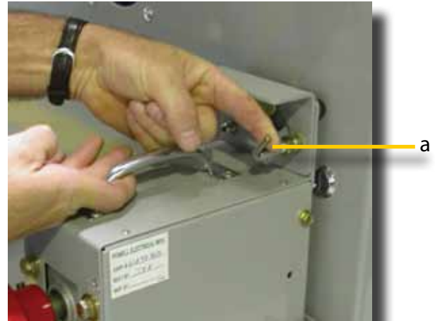
Figure 19 Turn the Spring Lock Pin to Secure the Racking Device on the Support Lock Pin
