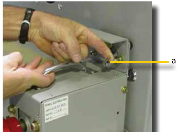
Figure 11 Turn the Spring Lock Pin to Secure the Racking Device on the Support Lock Pin
